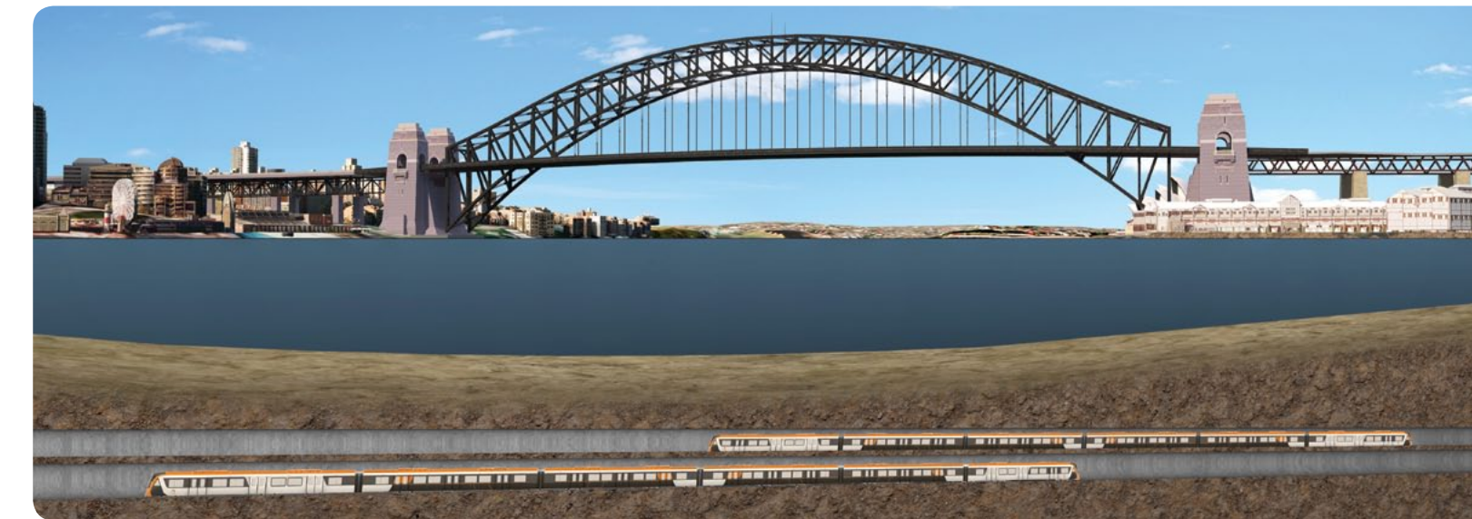
Rapid transit under Sydney Harbour.
